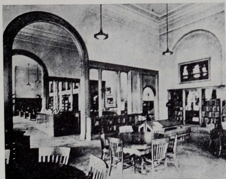
Pl. II. — Carpenter Branch Library, St-Louis.
